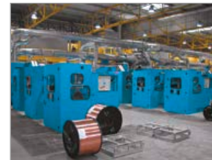
Exhaust air systems
